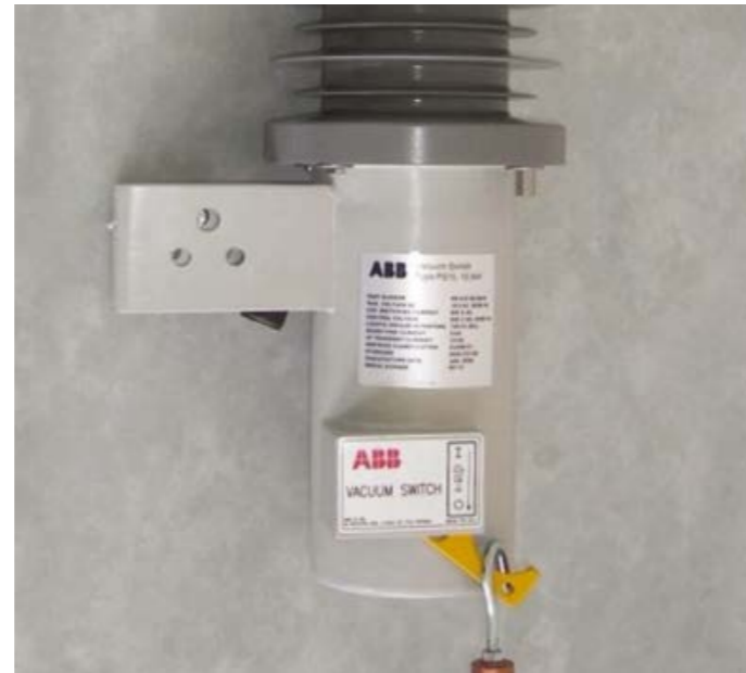
Figure 5b: OPEN switch using hook stick
